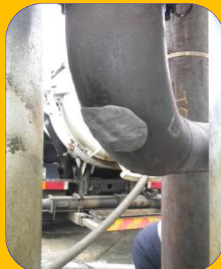
1. F.S. STEEL EPOXY
