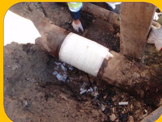
6. COMMISSIONING 2H AFTER
