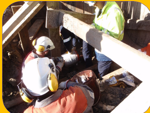
4. RECOVERY WITH BANDE PR
