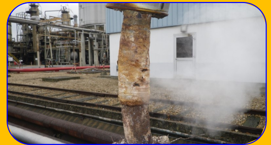
LEAK APPEARED AFTER 47 MONTHS IN SERVICE JANUARY 2014
