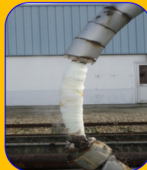
JANUARY 2014 RECOVERING WITH : Ruban RS-HT + Bande PR
