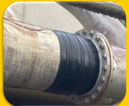
**LIGNE SECTIONNÉE - ÉCOULEMENT D'EAU + VAPEUR - APPLICATION EN CHARGE**
